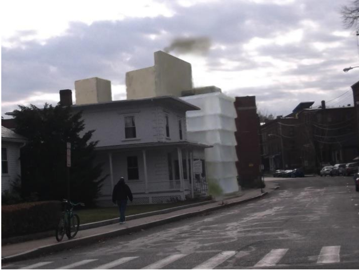
60 Masonic Street, Northampton MA
